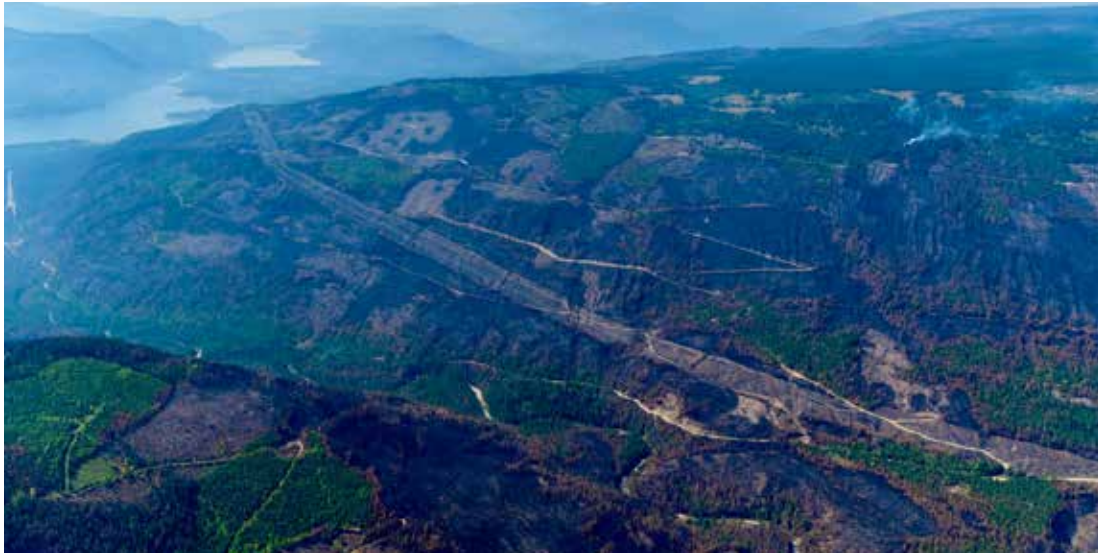
Location 1 top left where the power line turns to the right
